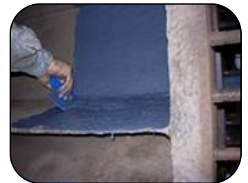
Process vessel surfaces badly corroded from chemical attack rebuilt using PES 201 Ceramic Repair Paste
