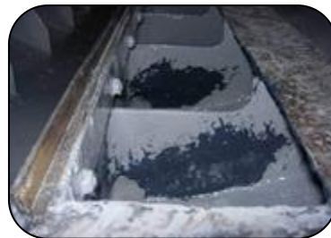
Process vessel surfaces badly corroded from chemical attack rebuilt using PES 201 Ceramic Repair Paste
