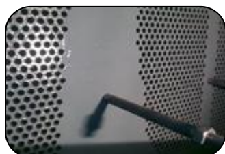
Condenser tube sheet resurfaced
