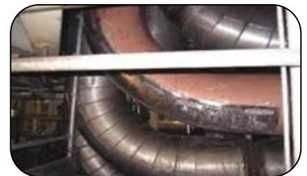
Coal lines at a power station rebuilt and protected using PES 204 Heavy Duty Ceramic Repair Paste
