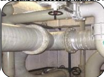
Main fire water lines encapsulated using PES 301 Epoxy Resin and Hardener and 3 wraps of Glass Tape
