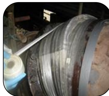
Eroded gas main repaired using PES 301 Epoxy Resin and Hardener and 3 wraps of Glass Tape
