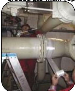
Main fire water lines encapsulated using PES 301 Epoxy Resin and Hardener and 3 wraps of Glass Tape
