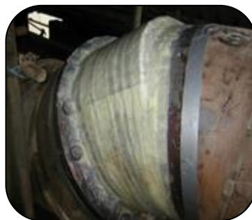
Eroded gas main repaired using PES 301 Epoxy Resin and Hardener and 3 wraps of Glass Tape
