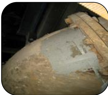
Eroded gas main repaired using PES 301 Epoxy Resin and Hardener and 3 wraps of Glass Tape
