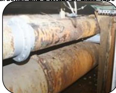
Main fire water lines encapsulated using PES 301 Epoxy Resin and Hardener and 3 wraps of Glass Tape
