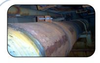
1000s of feet pipework completed on board vessels worldwide manual surface prep with three wraps of glass tape and 301 Epoxy Resin and Hardener.
